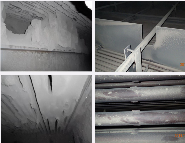
Visual results before (left) and after (right) preventive cleaning with Infrasound Technology
